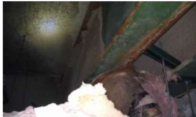
Cavity between the floor of the Recreation Yard and ceilings below.
